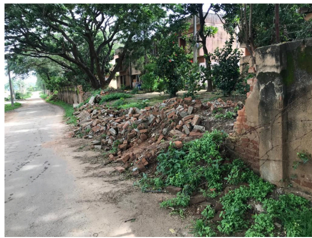
Photo of Collapsed Wall at Officers' Quarters :
