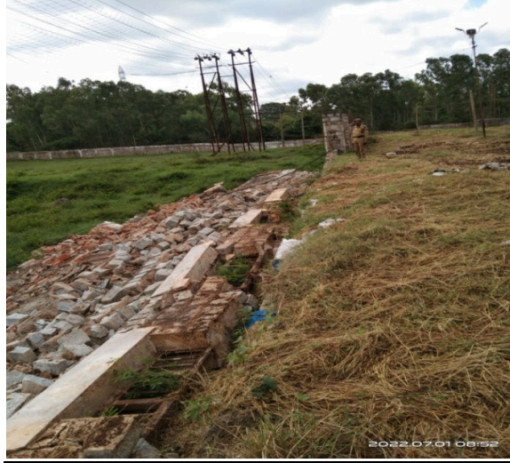
Photo of Collapsed Wall at Tower-4 at EM Division :
