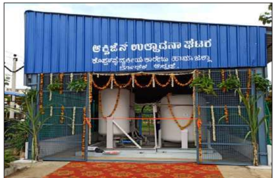
Medical Oxygen Plant
