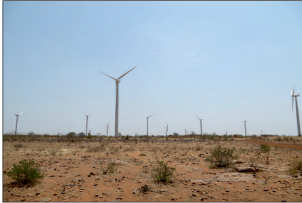
A view of BEML Windmill Project
