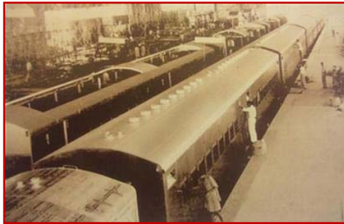
Metal Rail Manufacturing facility
